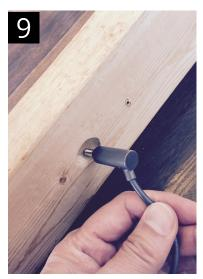
Push the tip of the charging cord (or jack plug) through the hole.
