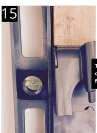
Check the wood post is vertical by using a spirit level.
