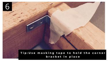
On the other side of the 2x4 horizontal stud post, position the corner bracket. Do not align with the corner bracket on the other side.
