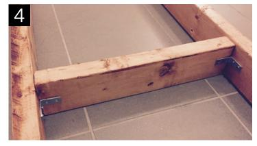
Position the horizontal stud post between the vertical posts and centre on corner brackets.
