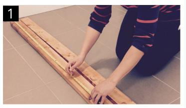
Lay both vertical stud posts flat on the floor side by side. Measure half way up each stud post and mark a spot in the centre.
