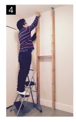
Turn the adjusting screws clockwise to tighten.
