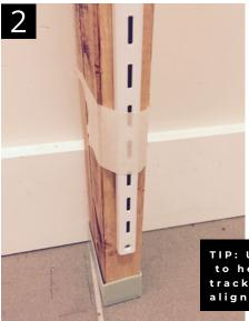
Align the mark with the bottom hole of the 48" shelf track.
