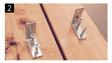
Place corner bracket over the marked spot and align with the bottom screw hole. Drill pilot holes then screw into the timber using 1 ¼' screws.
