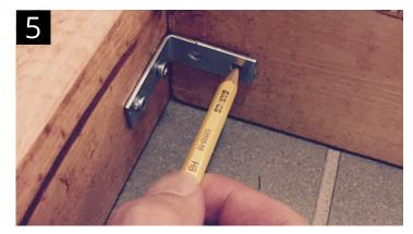
Mark the screw holes and drill pilot holes. Fasten the bracket to the studusing 1  $\frac{1}{4}$  screws.
